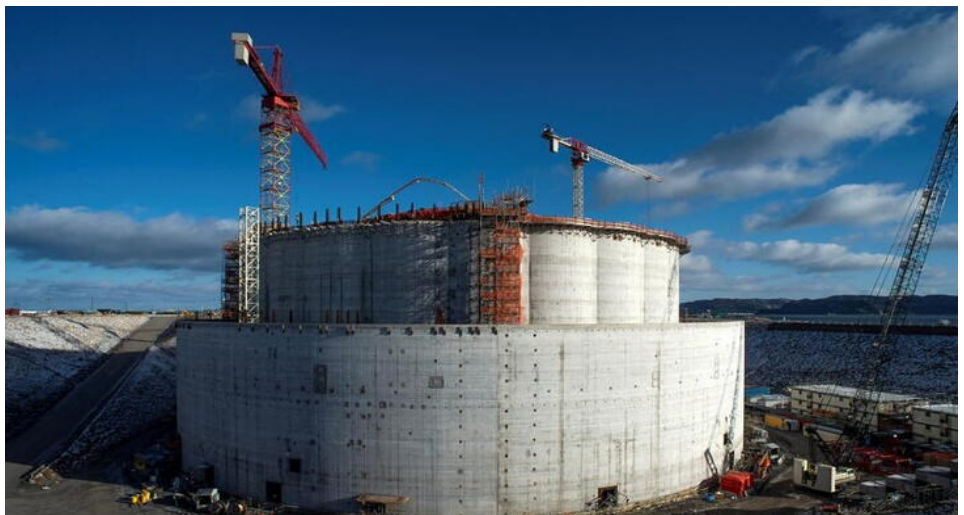
The fixed wellhead platform of Cenovus Energy's West White Rose extension project is seen under construction in Argentia, Placentia Bay, Newfoundland, December 13, 2019. REUTERS/Greg Locke
