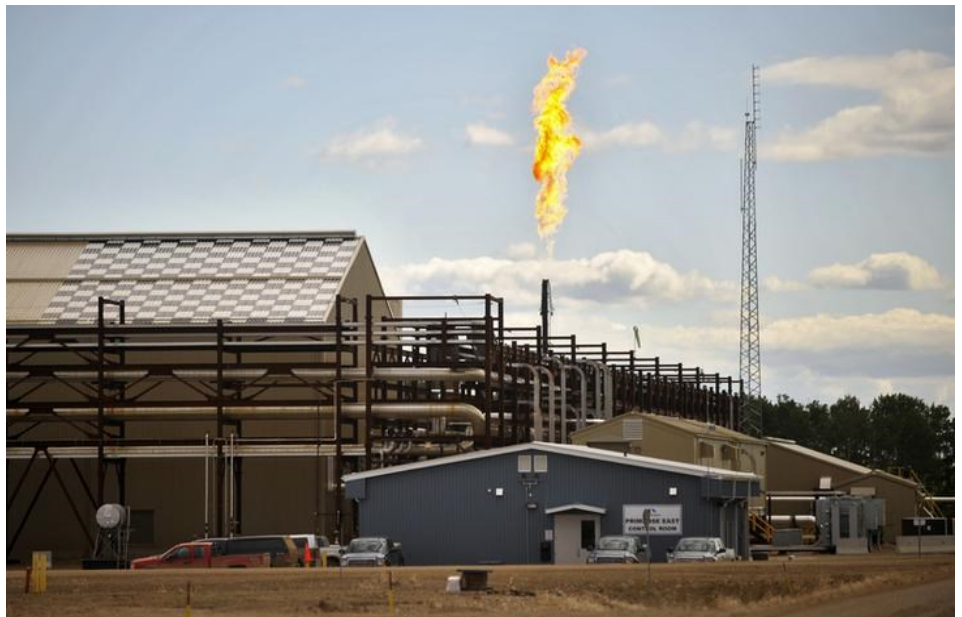
The suspension of steam generation forces this East Primrose steam plant to flare natural gas at Canadian Natural Resources Limited's Primrose Lake oil sands project near Cold Lake, Alberta, August 8, 2013. REUTERS/Dan Riedlhuber
