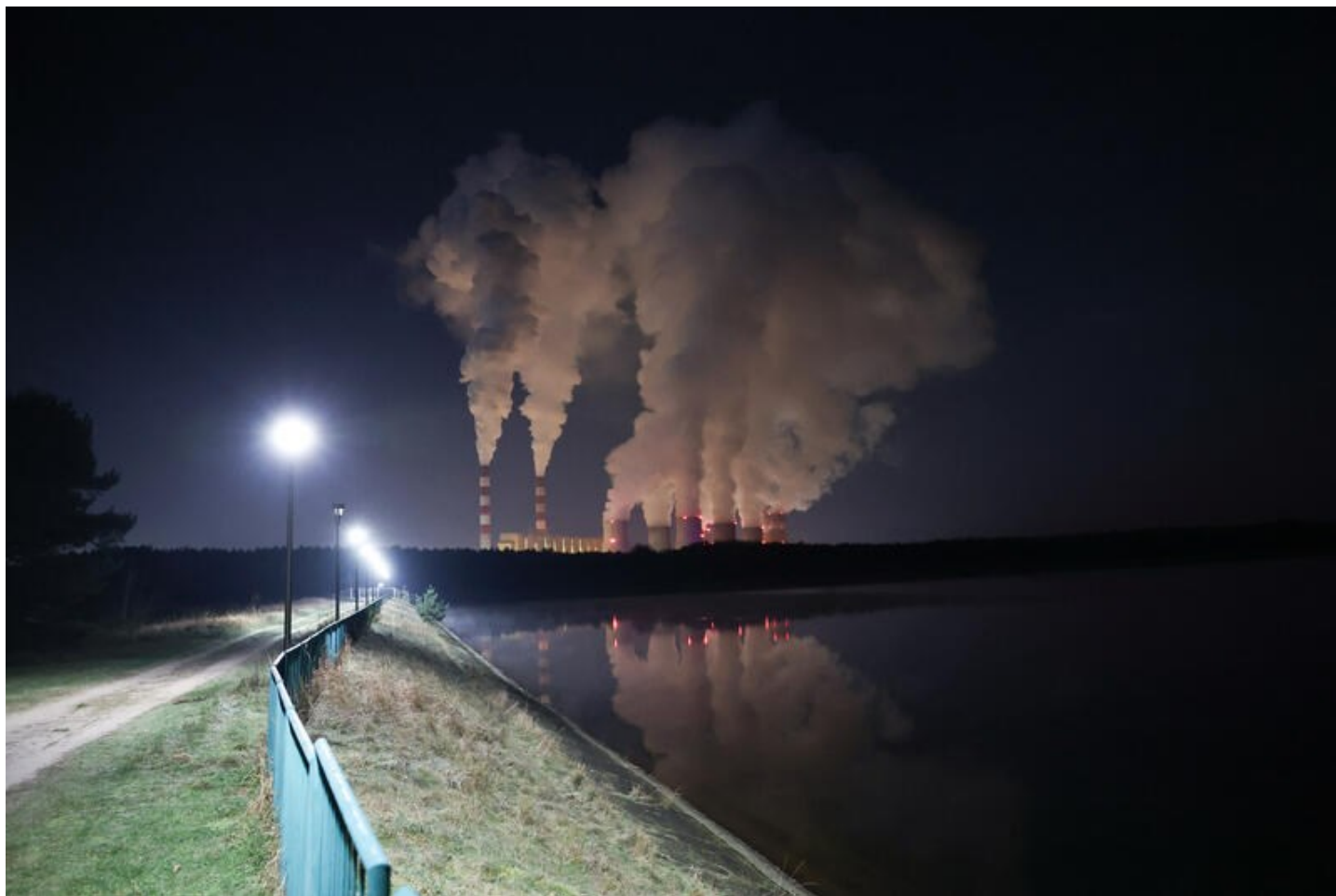
Smoke and steam billow from Belchatow Power Station, Europe's largest coal-fired power plant powered by lignite, operated by Polish utility PGE, at night in Rogowiec, Poland, November 22. REUTERS/Kacper Pempel
