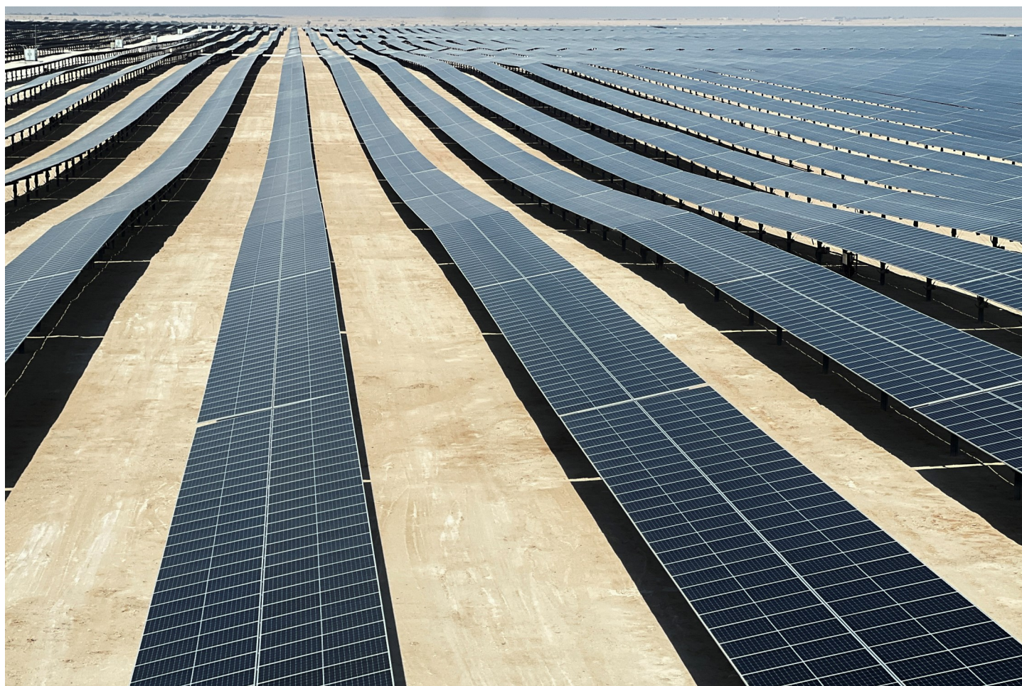
Solar Panels are seen at the Al Kharsaah solar plant project, in Al Kharsaah, Qatar. REUTERS/Imad Creidi
