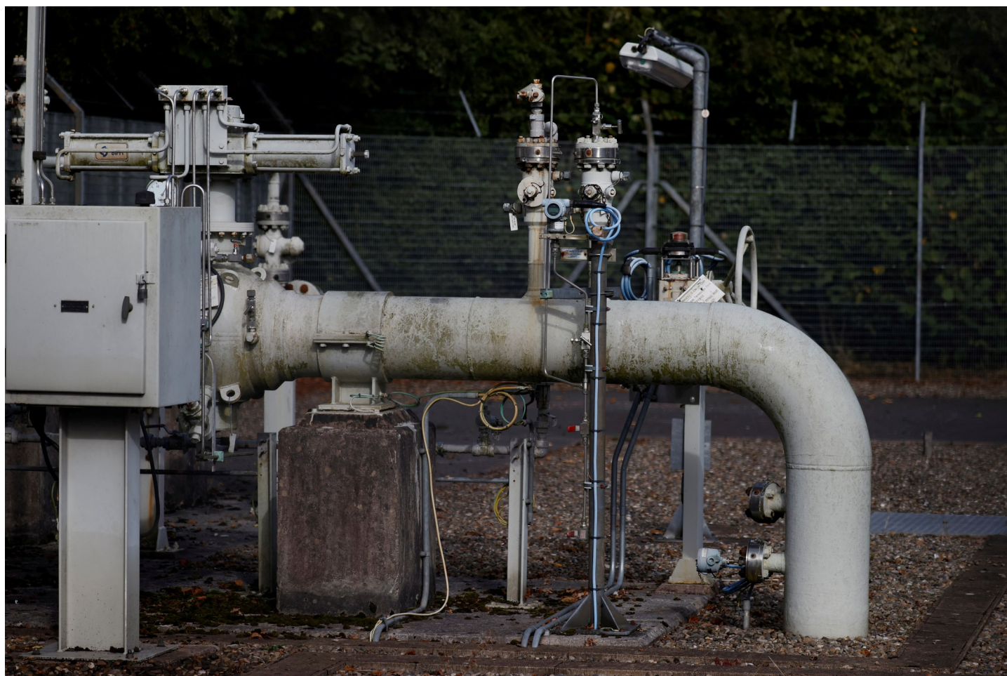
A section of gas pipeline is seen at a National Grid facility near Knutsford, Britain. REUTERS/Phil Noble
