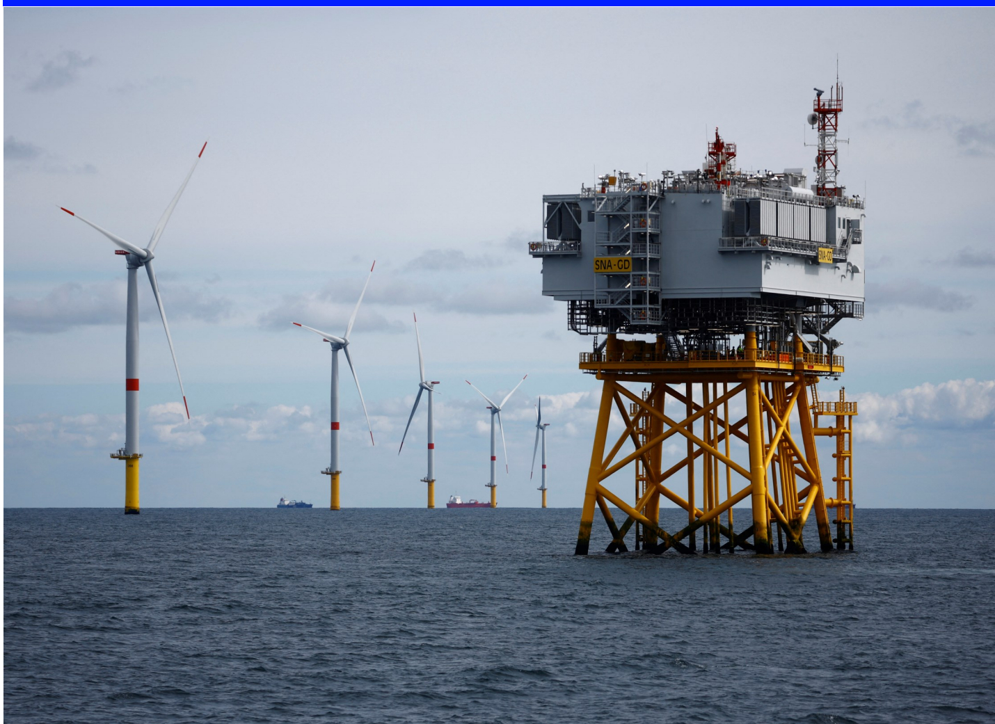
Wind turbines are seen at the Saint-Nazaire offshore wind farm, off the coast of the Guerande peninsula in western France. REUTERS/Stephane Mahe
