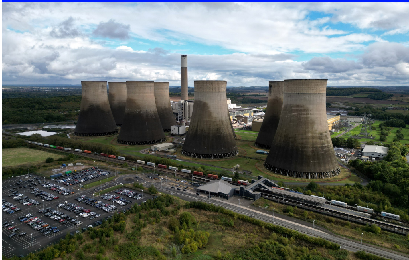
A drone view of Ratcliffe-on-Soar Power Station in Ratcliffe-on-Soar, Nottinghamshire, Britain, September 26. REUTERS/Molly Darlington
