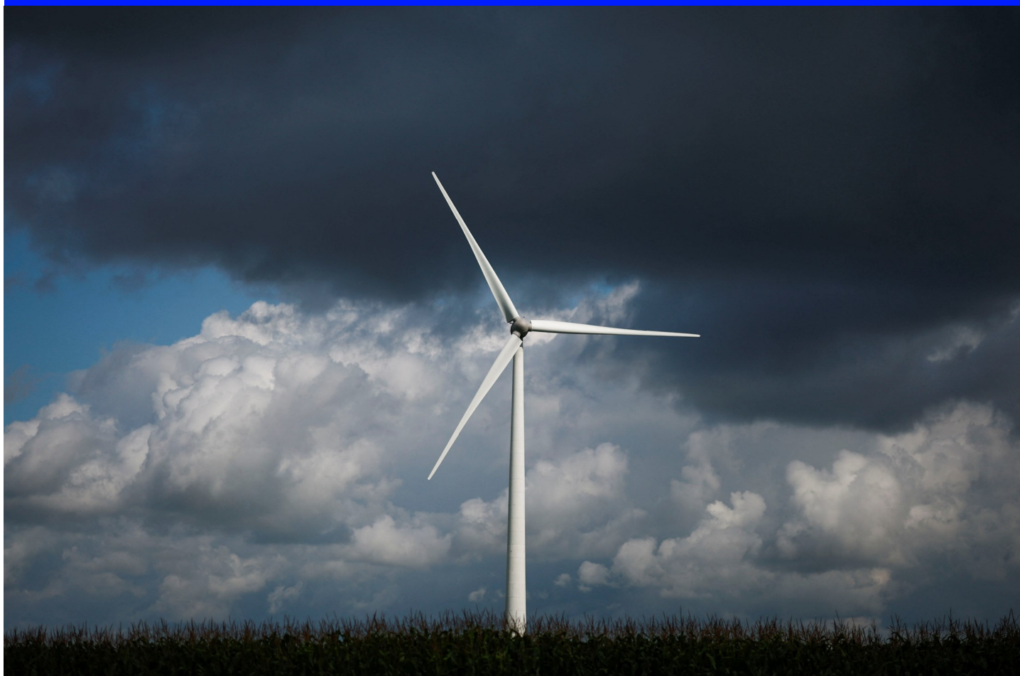
A view shows a power-generating windmill turbine at a wind park in Ligne near Nantes, France, September 23. REUTERS/Stephane Mahe
