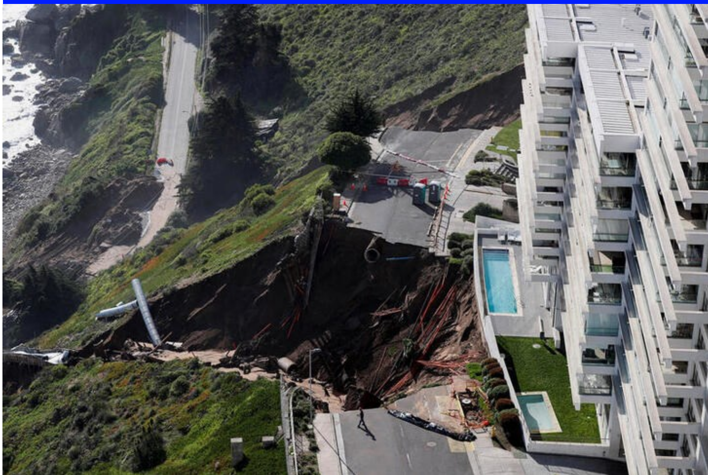
View of a massive landslide next to a building complex, after heavy rains hit Concon, Chile, September 11. REUTERS/Rodrigo Garrido
