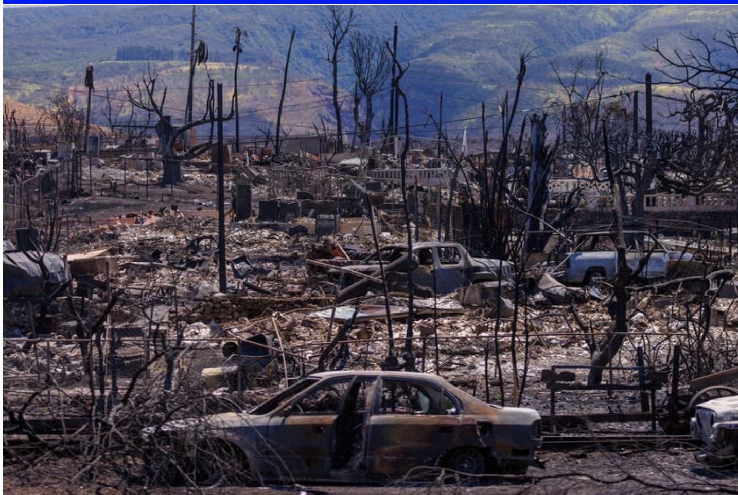
Fire damage is shown in the Wahikuli Terrace neighborhood in the fire ravaged town of Lahaina on the island of Maui in Hawaii, U.S., August 15, 2023. REUTERS/Mike Blake
