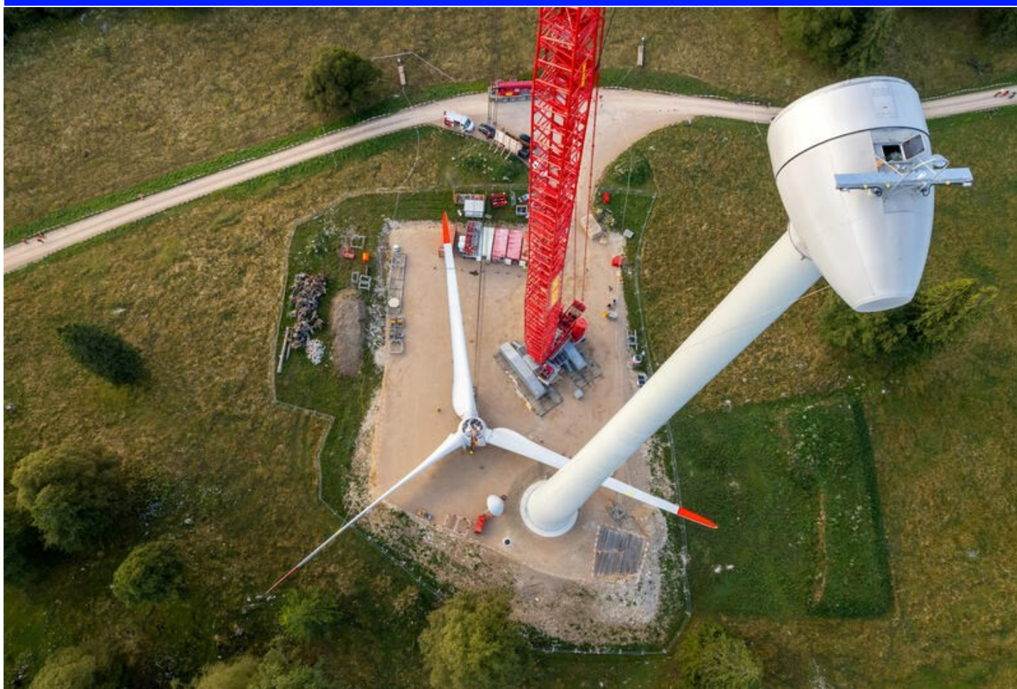
A crane of Enercon lifts a full hub consisting of three blades and the rotor for a wind turbine for Romande Energie in Ste-Croix, Switzerland, July 31, 2023. REUTERS/Denis Balibouse
