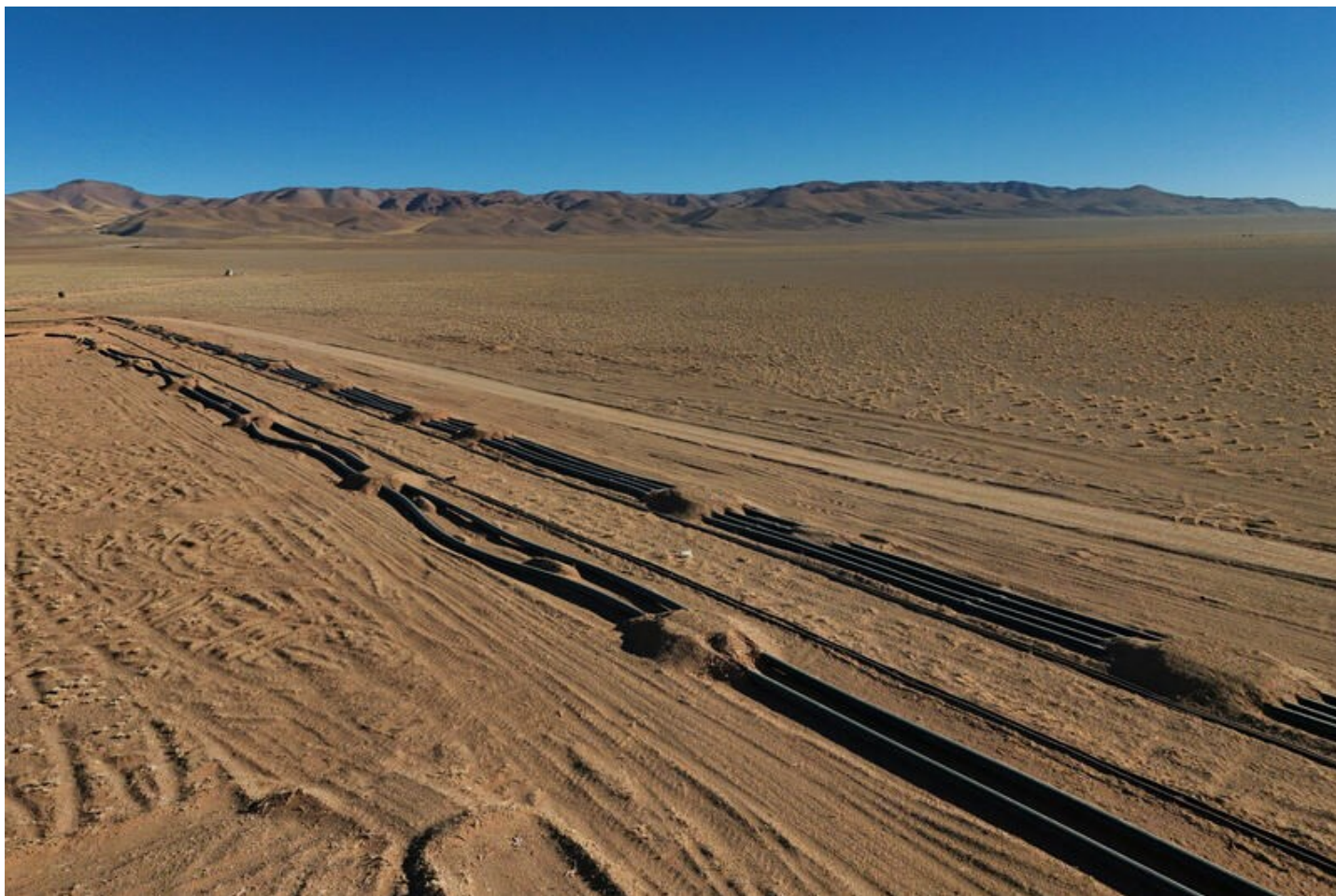
A drone view shows brine transport pipes at the Eramet's lithium production plant at Salar Centenario in Salta, Argentina July 4. REUTERS/Matias Baglietto
