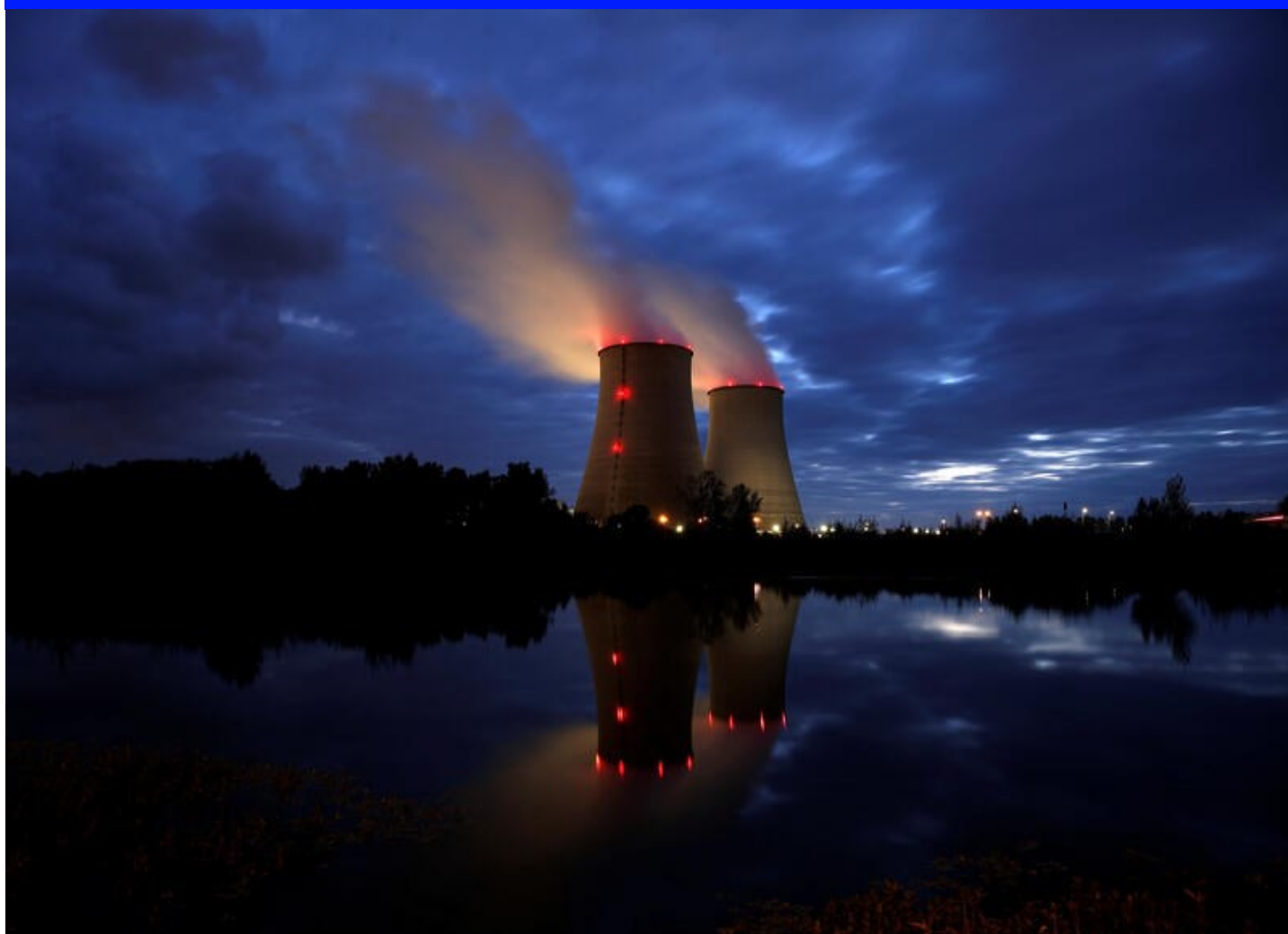
Steam rises from cooling towers of the Electricite de France (EDF) nuclear power plant in Belleville-sur-Loire. REUTERS/Benoit Tessier
