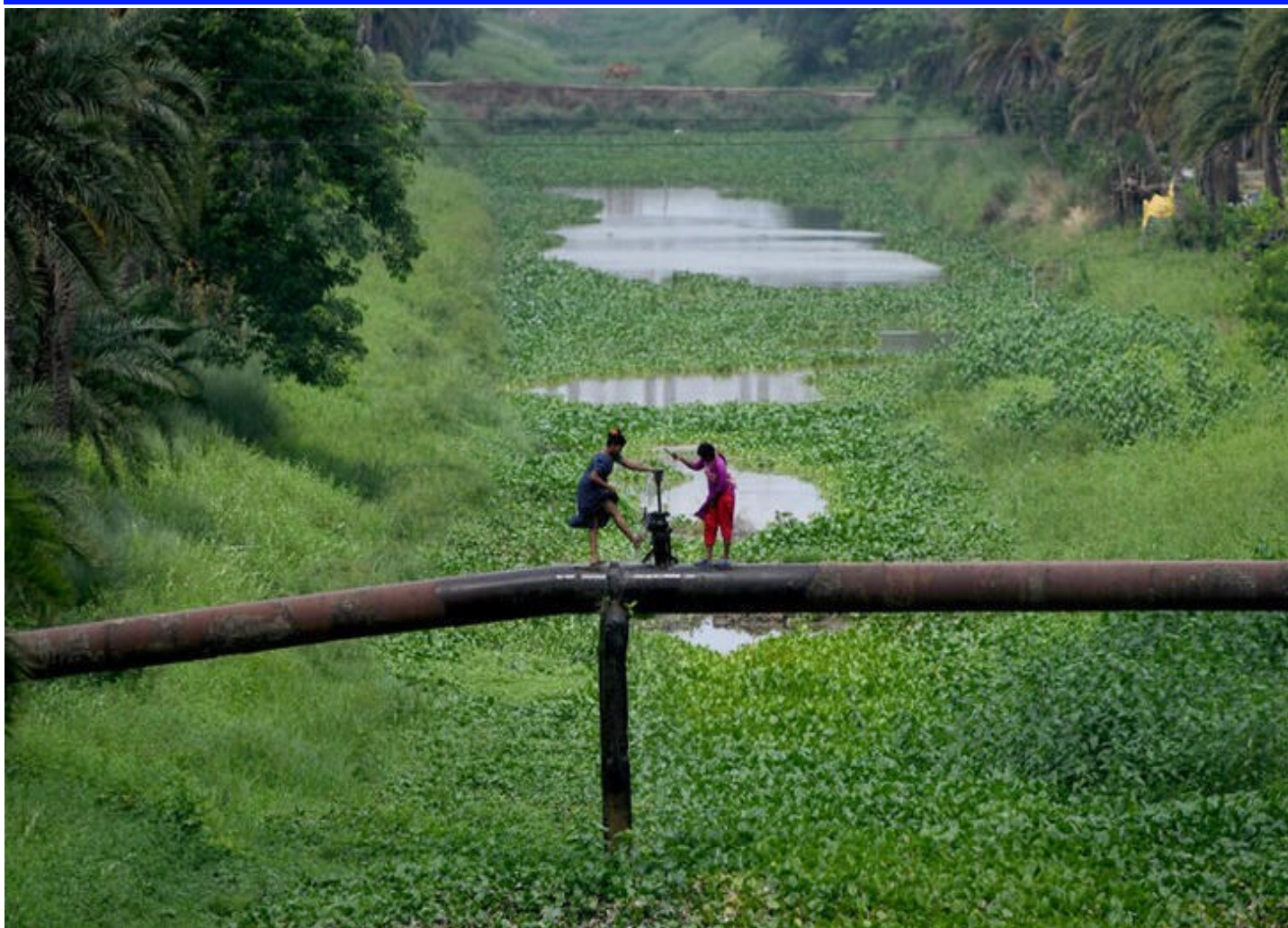
Women wash their feet from a leaked valve of a water pipe laid across a canal in Kendrapara district in the eastern state of Odisha, India, May 30. REUTERS/Stringer
