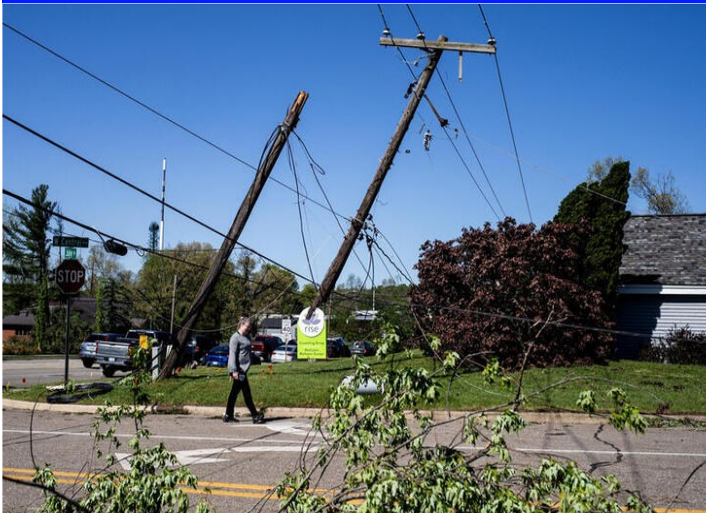
A resident walks past downed electrical lines after a tornado hit the area of Portage, Michigan, U.S., May 8. REUTERS/Emily Elconin
