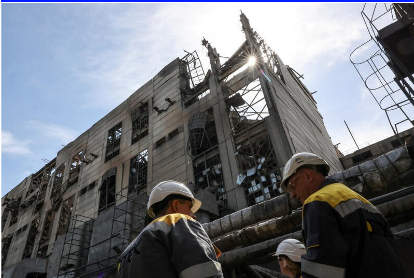
Thermal power plant employees appear on site at the building damaged by recent Russian missile strikes, amid Russia's attack on Ukraine, at an undisclosed location in the west of Ukraine, May 2. REUTERS/Roman Baluk
