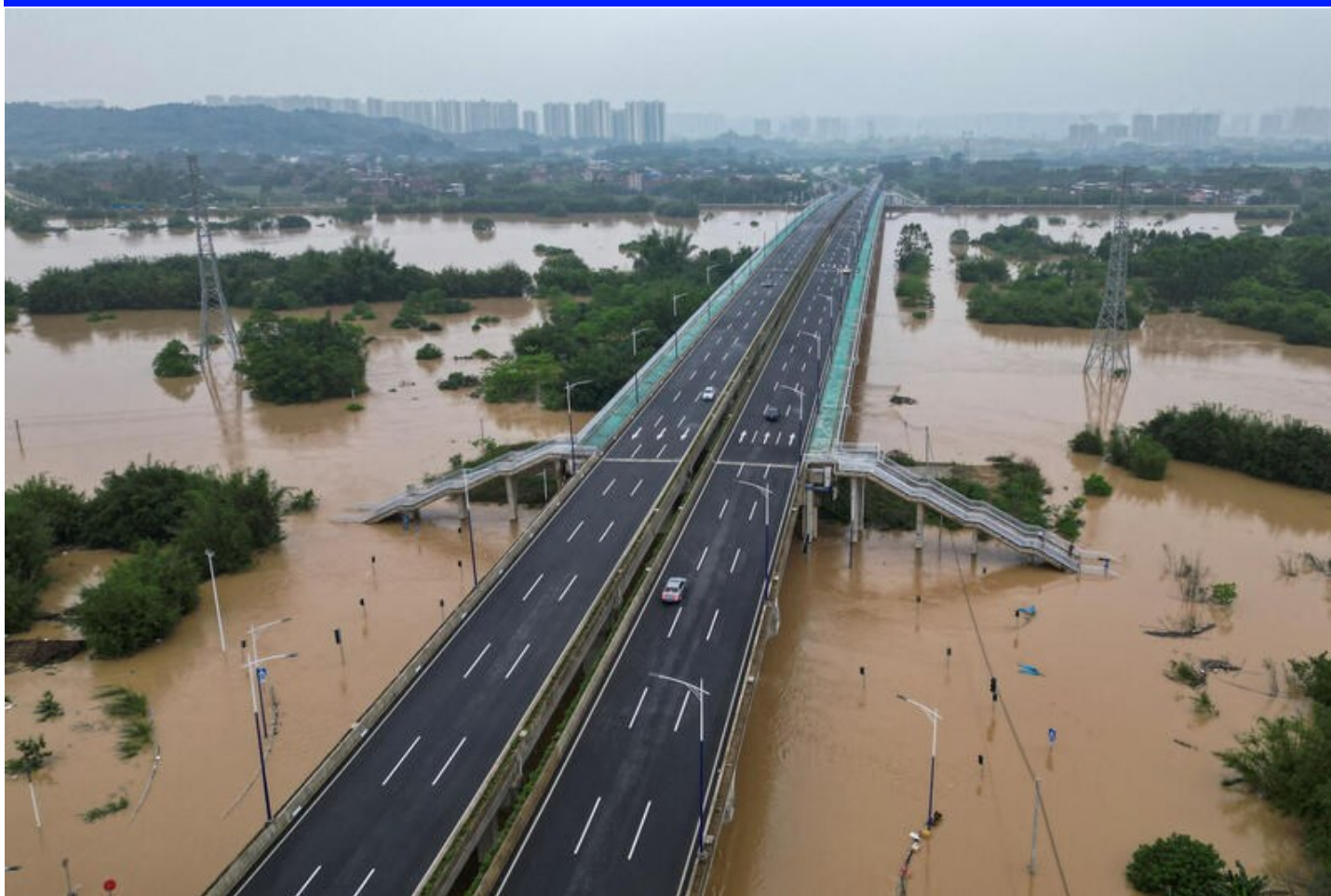
A drone view shows roads submerged in floodwaters following heavy rainfall, in Qingyuan, Guangdong province, China April 22, 2024. REUTERS/Tingshu Wang
