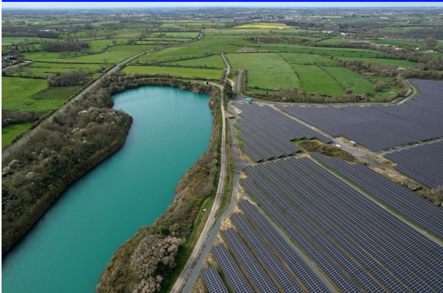
A drone view shows solar panels at a photovoltaic park in Sevreinoie near Cholet, France, March 25. REUTERS/Stephane Mahe
