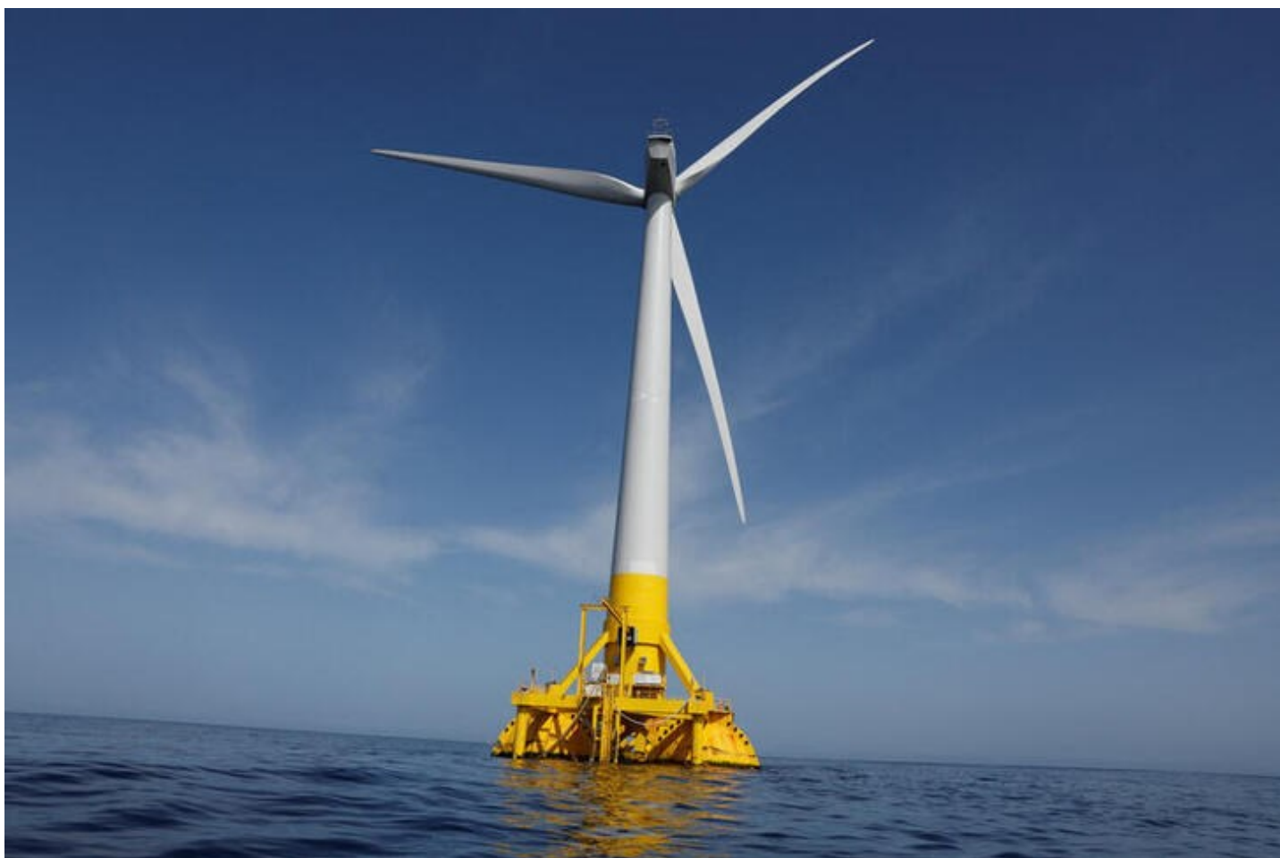
An experimental offshore wind turbine manufactured by Spanish company Saitec operates near the coastal town of Armintza, Spain, March 21. REUTERS/Vincent West
