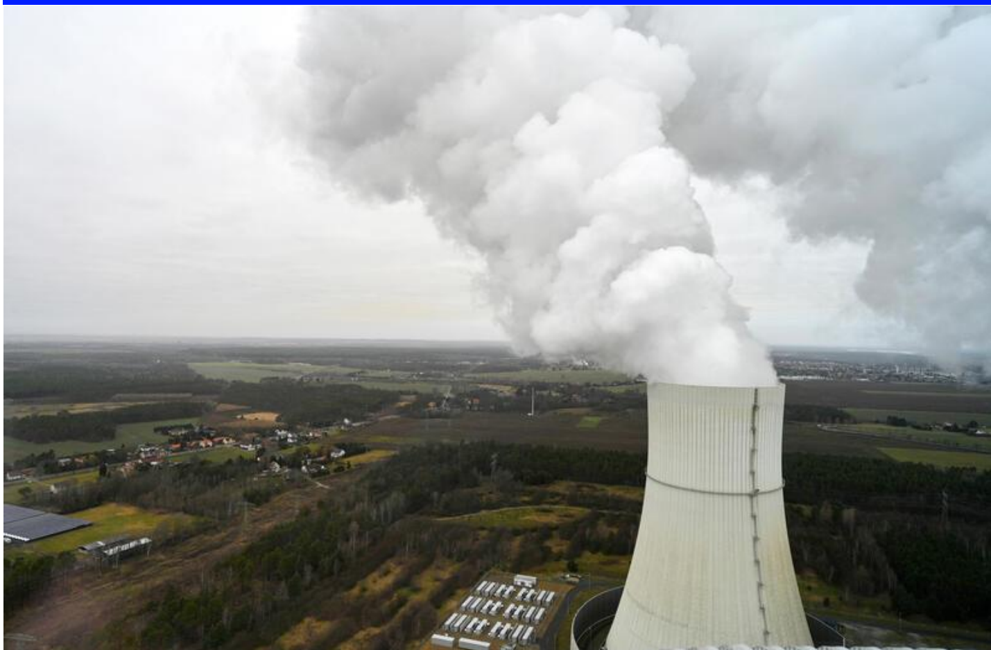
A general view of Schwarze Pumpe power plant of company LEAG, in Spremberg, Germany, February 22. REUTERS/Matthias Rietschel
