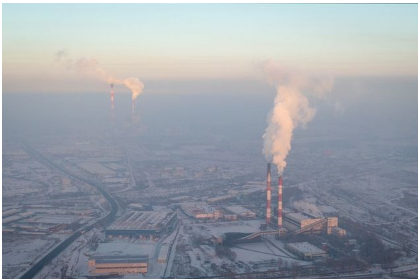
An aerial view shows a thermal power plant in the Siberian city of Krasnoyarsk, Russia, February 12. REUTERS/Alexander Manzyuk
