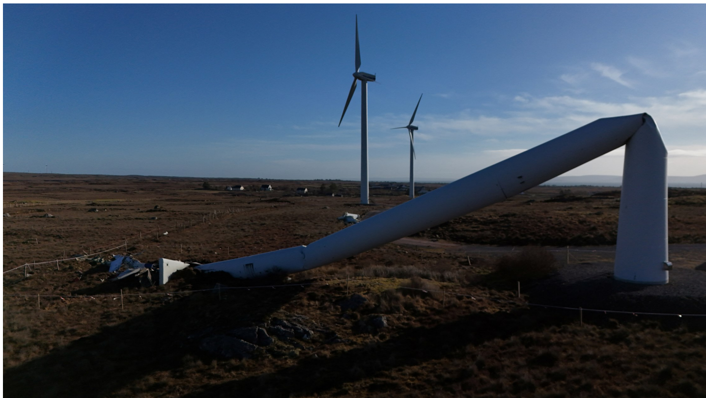
A drone view shows a damaged wind turbine that was blown over during Storm Eowyn, in Inverin, Ireland, January 29. REUTERS/Clodagh Kilcoyne
