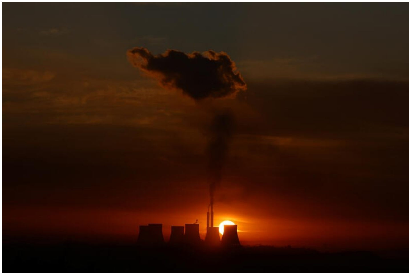
The sun rises behind the cooling towers of Kendal Power Station, a coal-fired station of South African utility Eskom, as the company's ageing coal-fired plants cause frequent power outages, near Witbank, in the Mpumalanga province, South Africa, 2023. REUTERS/
