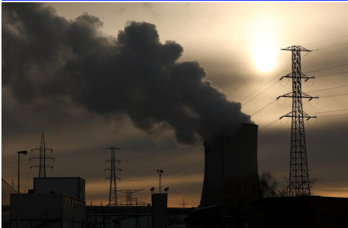
Smoke billows from a chimney at a combined-cycle gas turbine power plant in Drogenbos, Belgium, January 16. REUTERS/Yves Herman
