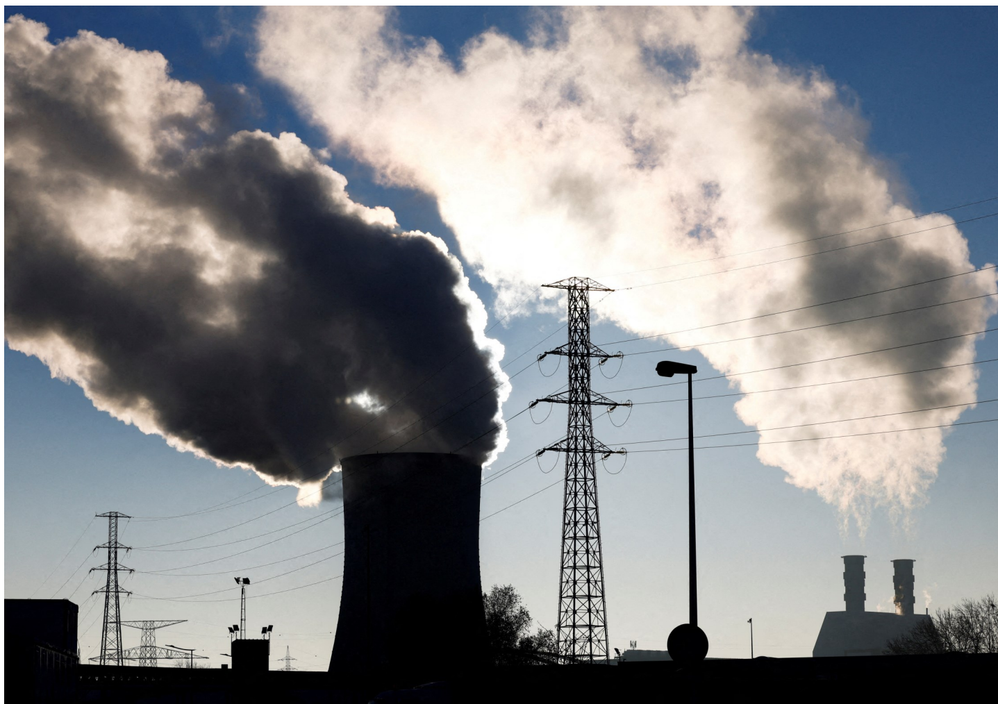
Electric pylons are seen at an Engie subsidiary Electrabel combined-cycle gas turbine power plant in Drogenbos, Belgium. REUTERS/Yves Herman
