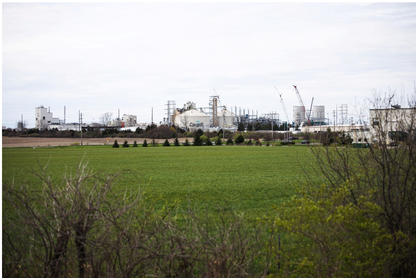
Storage tanks are seen at the Cargill Inc soybean processing facility in Sidney, Ohio, U.S.. REUTERS/Megan Jelinger
