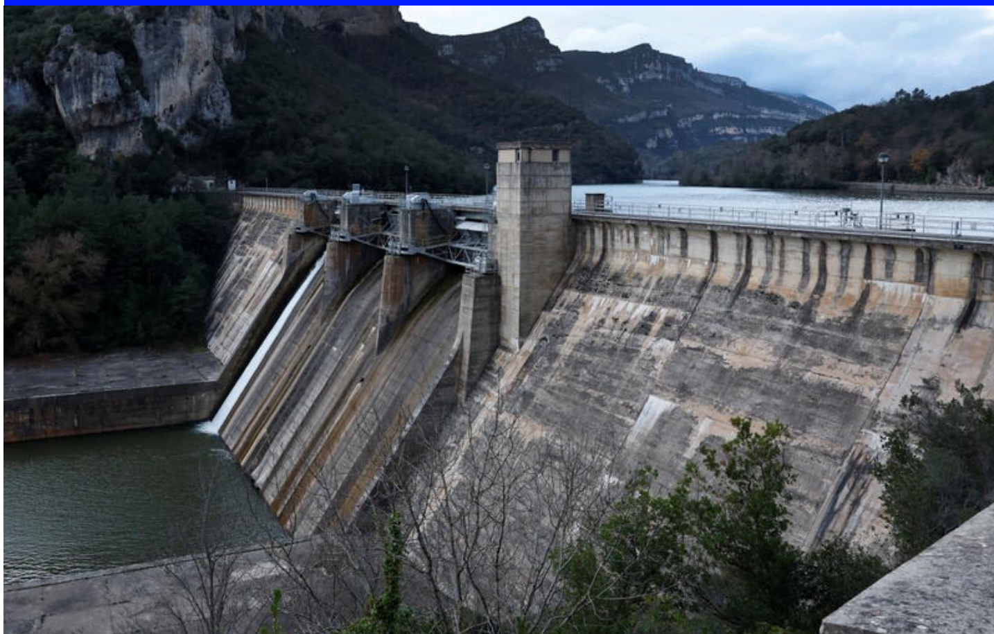
A view shows Sobron hydroelectric dam on the Ebro River, in Burgos province, Spain, January 4. REUTERS/Vincent West
