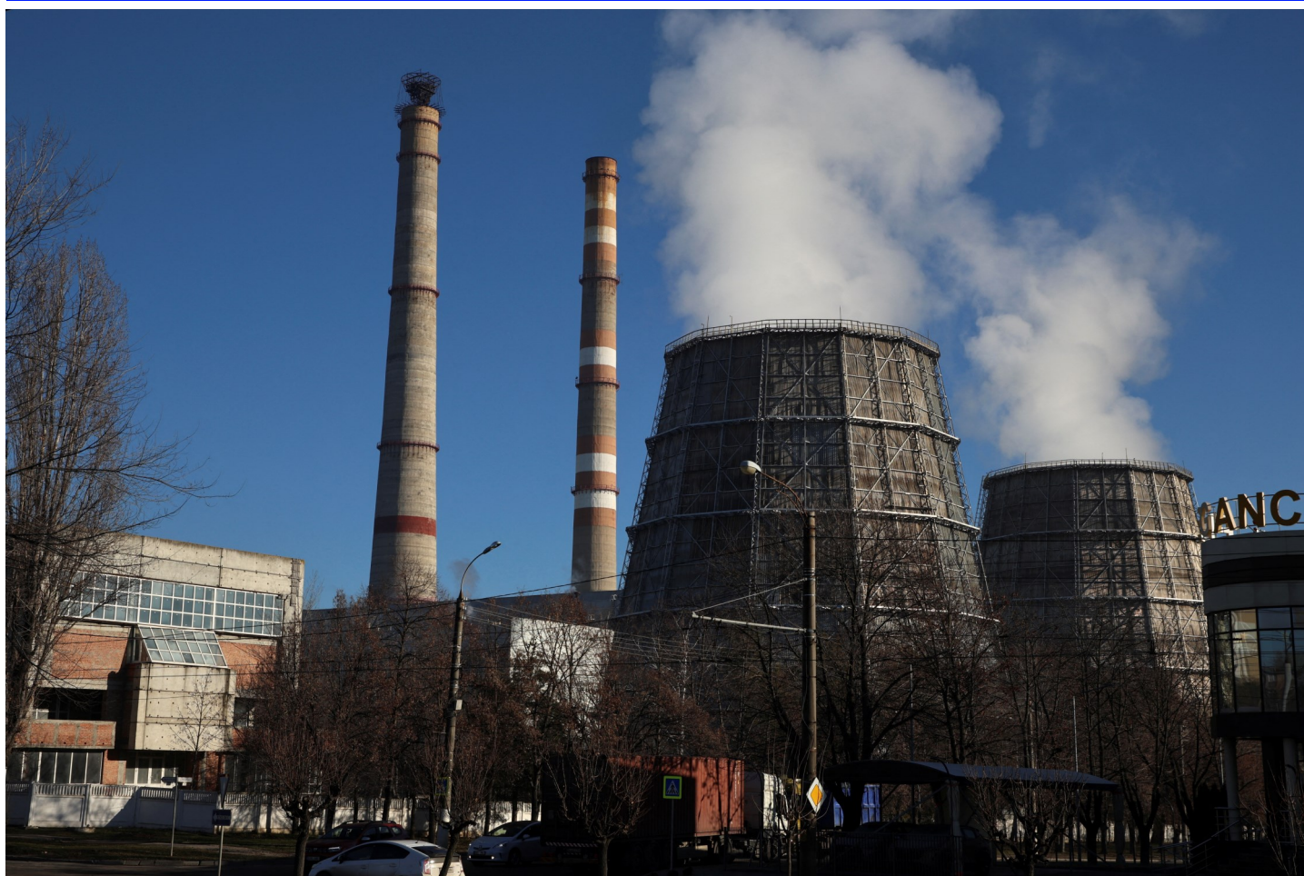
A view shows a thermal power station in Chisinau, Moldova, December 31. REUTERS/Vladislav Culiomza
